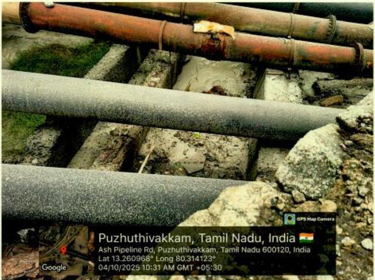
Same photo of ASDL line No. 3 welding joint
